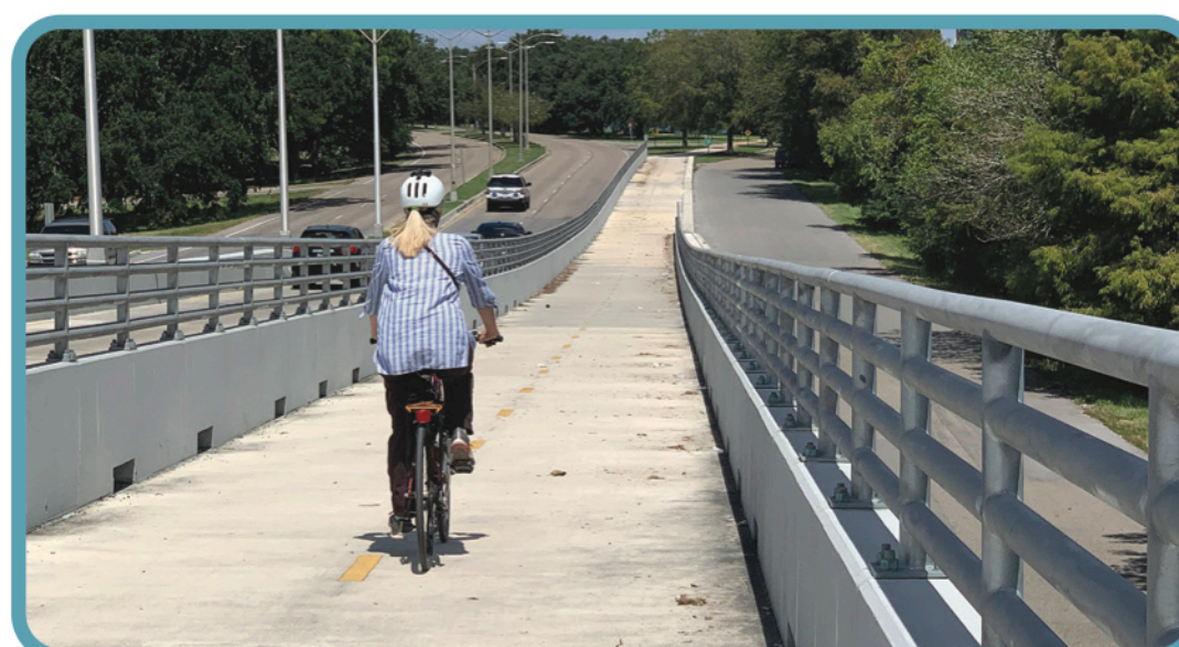
Wisner Bridge bicycle and pedestrian trail
