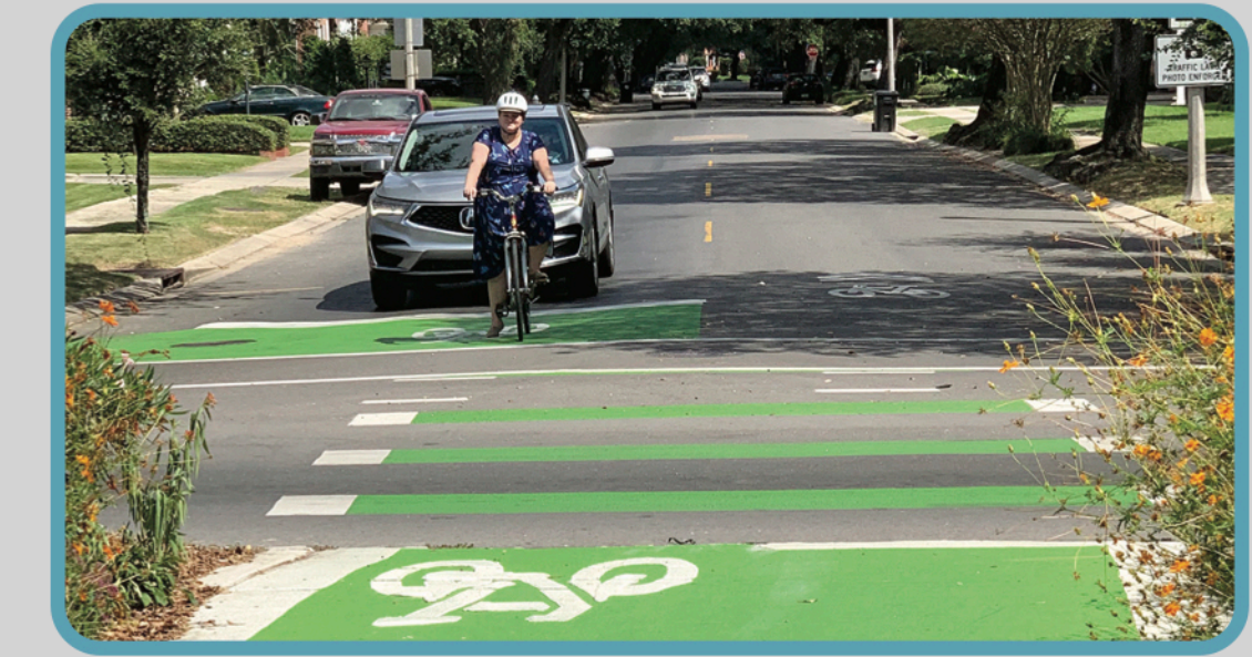
Vendome Place green bike box and median crossing
