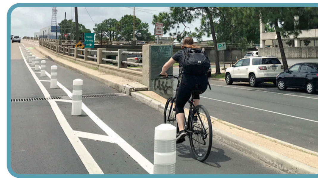
New protected lanes are being installed around the city to promote safety.
